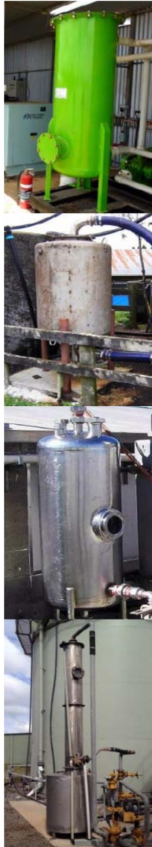
Fig 6 – Equipment used to encourage condensation by cooling the biogas and for collecting the condensate that forms before the biogas enters underground pipework.
