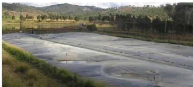
Figure 12 – Covered anaerobic pond (CAP) in Australia
