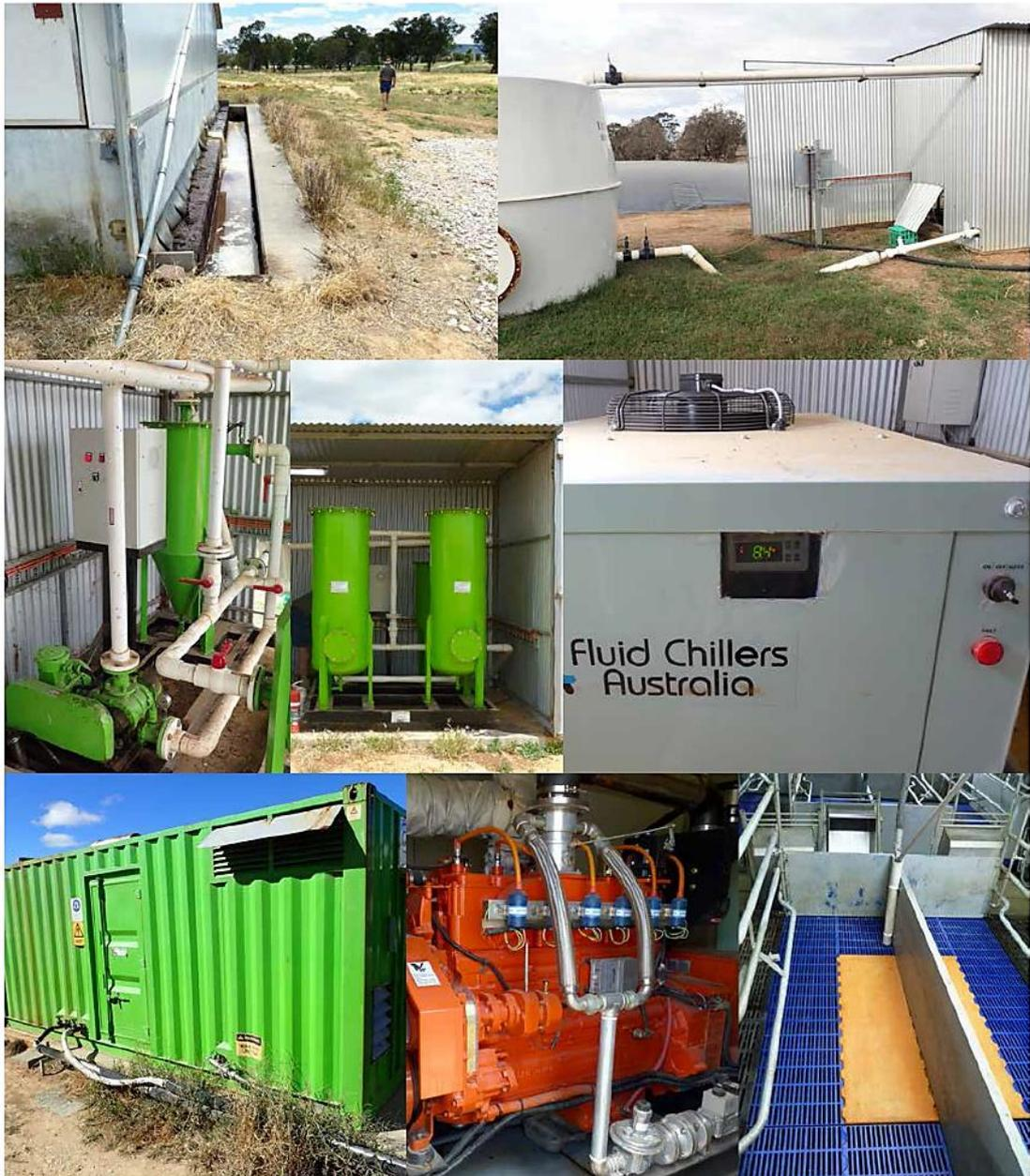
Figure 1: Biogas infrastructure at Pork CRC Demonstration Piggery 1
